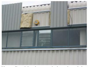
New rail and brackets attached on the existing wall cladding
