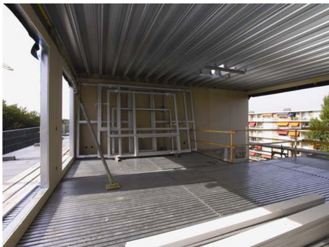
Figure 6 Light steel framework of roof-top extension in Rotterdam
