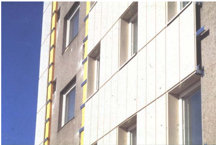
Figure 8 Over-cladding using light steel cassettes in Finland
