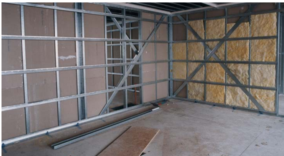
Figure 4 New light steel infill wall by Metsec for roof-top extension
