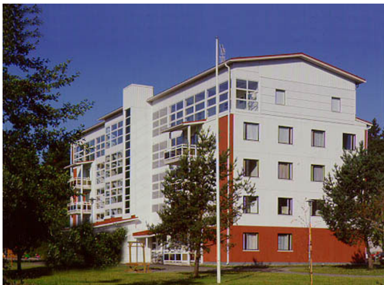
Figure 12 Modular units in roof-top extension in Finland
