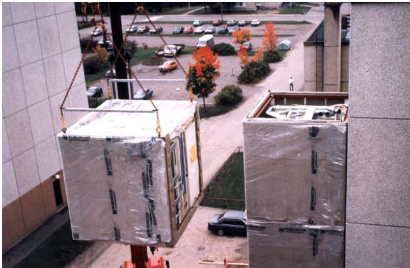
Figure 11 Toilet module in building extension in Finland (by Ruukki)
