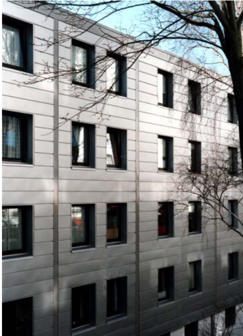
Figure 7 Over-cladding using horizontally orientated metallic panels
