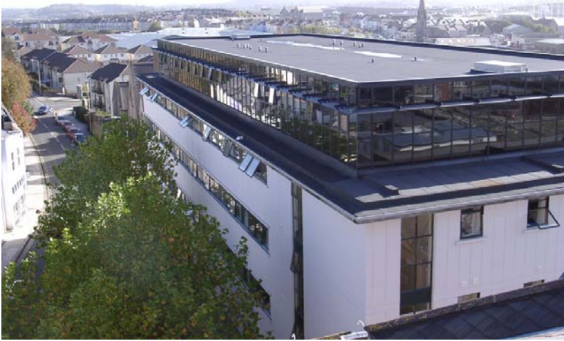
Figure 2 Roof-top extension of an existing building at Plymouth University
